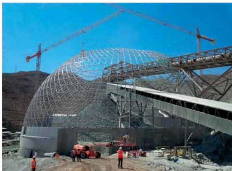
customization of the cladding panel on the dome allows for efficient and fast installation. The cladding panels were painted in order to add extra corrosion protection to the galvanized finish. The colour of the exterior and interior side of the panels matched client requirements.
