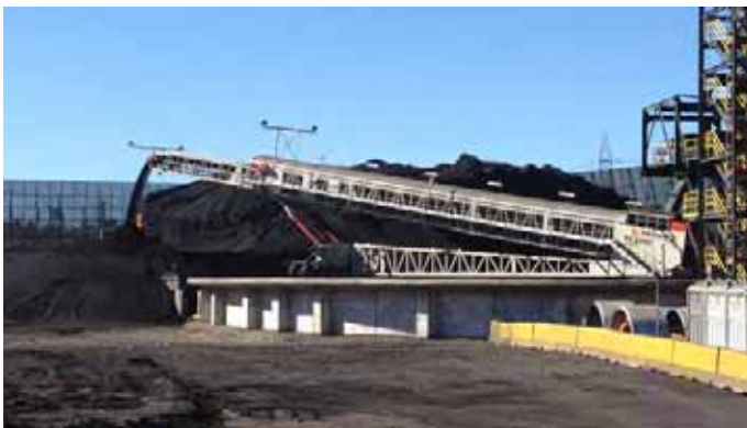
Radial Telescopic stockpiling coal @ 2000 TPH in powerplant
