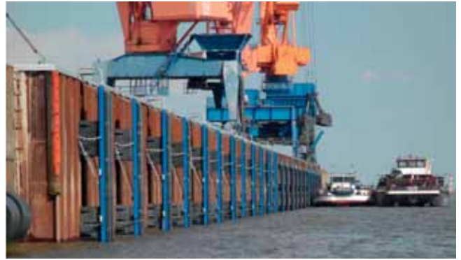
The new sheet pile wall in the middle berth in Brunsbüttel Elbe Port.
