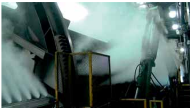
High density fog being projected into the dump pocket on the spillside of a rail dump hopper.
