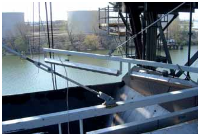
Nozzle boxes mounted on booms for access at barge unloading station.
