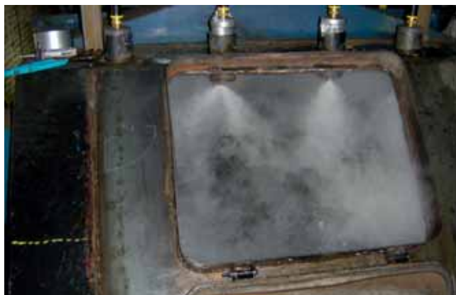
Nozzles operating in head box of tripper room conveyor. Note the fog follows the coal nicely into the chute allowing it to work on the dust as it becomes airborne.
