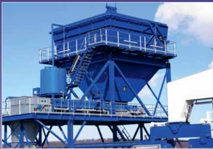
Hopper cars for ship unloading
