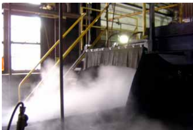
Tripper conveyor with 'tent'-type enclosure to allow belt lift. Fog follows the coal flow but filters all dust trying to escape the enclosure
