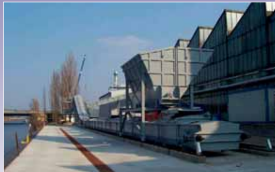
Conveying systems at the harbor
