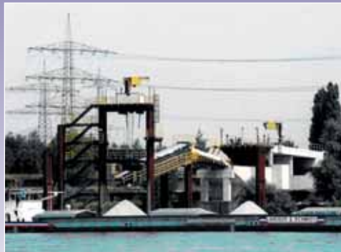
Ship loading systems
