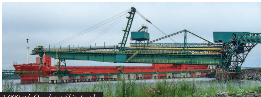
3,000 tph Quadrant Ship Loader
