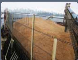
Fence incorporated with retaining wall
