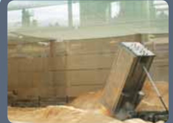
Fence with roof for easily blown dust
