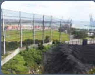
32m high fence for mountainside port storage
