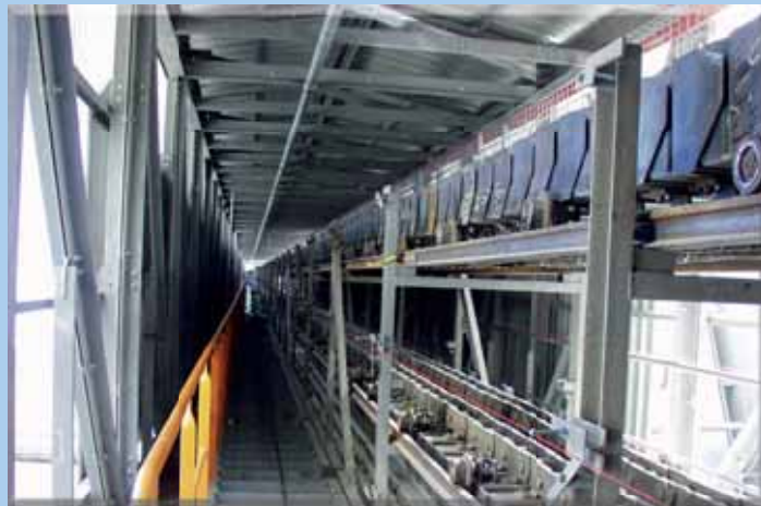
Clinker pan conveyor
