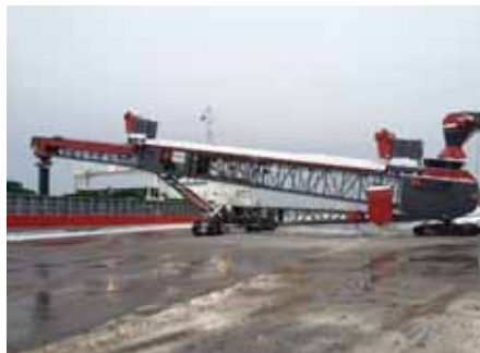
Telescopic shiploader with dust extraction & discharge chute, loading fertilizer in Baltics.
