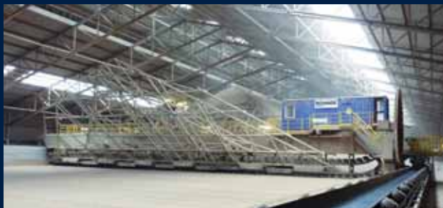
Bridge-type Reclaimer, wood pellets
