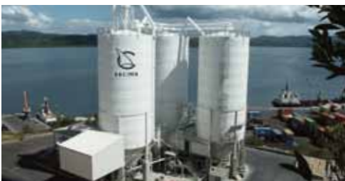
Terminal with steel silos for SACIMA, Port of Longoni, Mayotte Island, France
