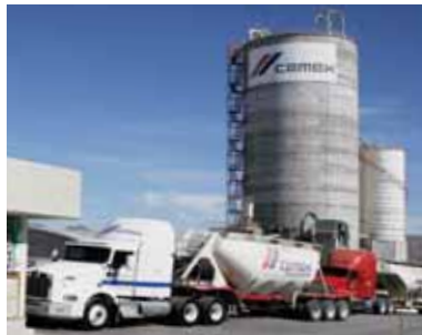
Cement import terminal for CEMEX, Mexico
