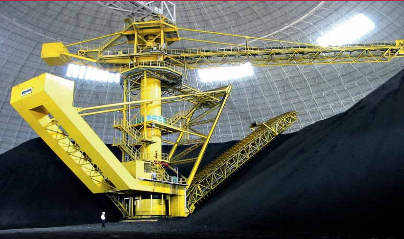
Circular Stockyard with Cantilever Reclaimer, coal
