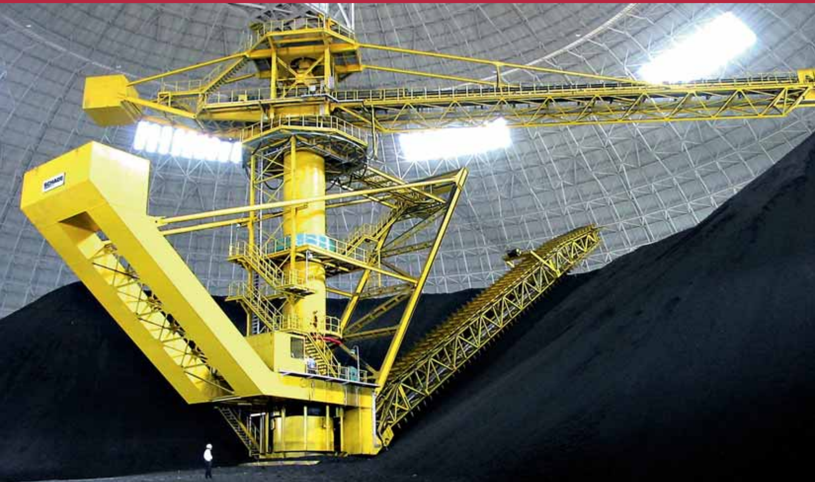
Circular Stockyard with Cantilever Reclaimer, coal
