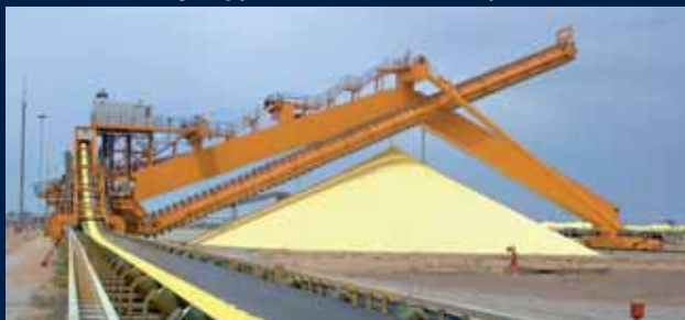
Combined Stacker / Reclaimer, sulphur prills
