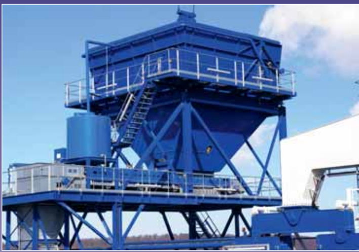
Hopper cars for ship unloading
