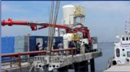
Jetty Mounted Ship Unloader
