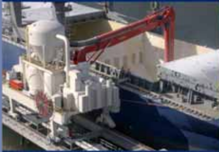
Rail Mounted Ship Unloader
