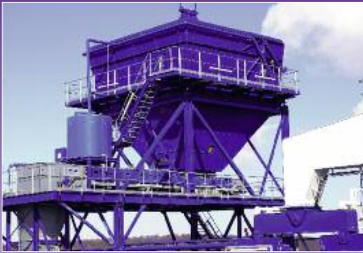
Hopper cars for ship unloading
