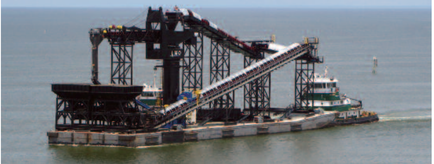
Featuring the "Louisiana Mid-Stream One", a unique barge-mounted conveying system that offers quality control features such as a metal collection and mechanical sampling.
