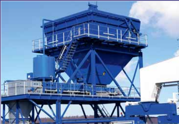
Hopper cars for ship unloading
