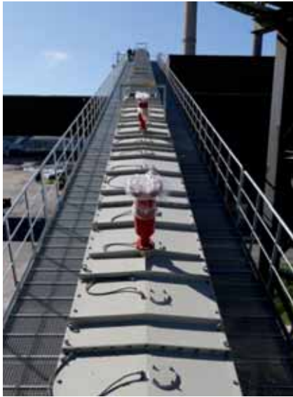
During the installation of an encapsulated trough chain conveyor belt system with modern explosion protection.
