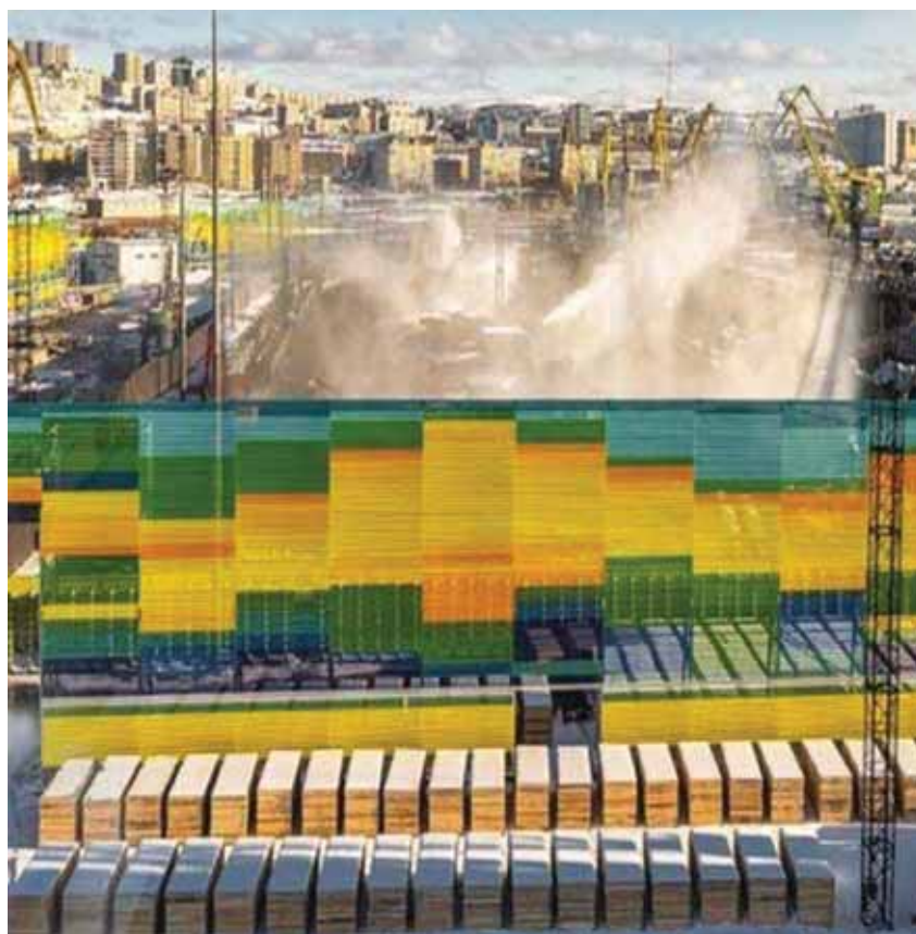
Dust-proof and wind-proof fences are used to combat dust in coal depots and port terminals.
