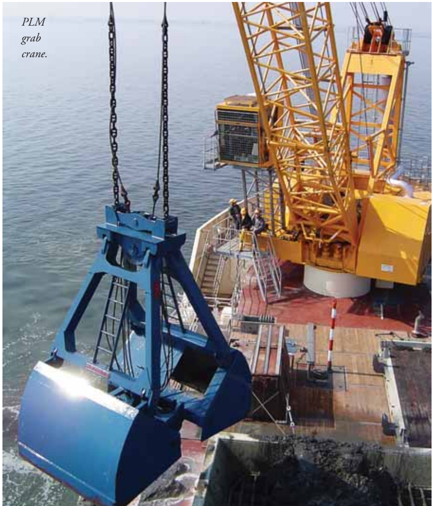
PLM offshore bulk handling crane.
