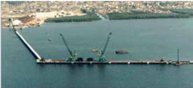
Two mobile travelling TMSA integrated solution with Manitowoc Cranes (USA) and TMSA (Brazil) mobile gantry and two aspirated hoppers with belt feeder, as well as 790m belt conveyor (2,000tph capacity) for a fertilizer import terminal in Brazil.
