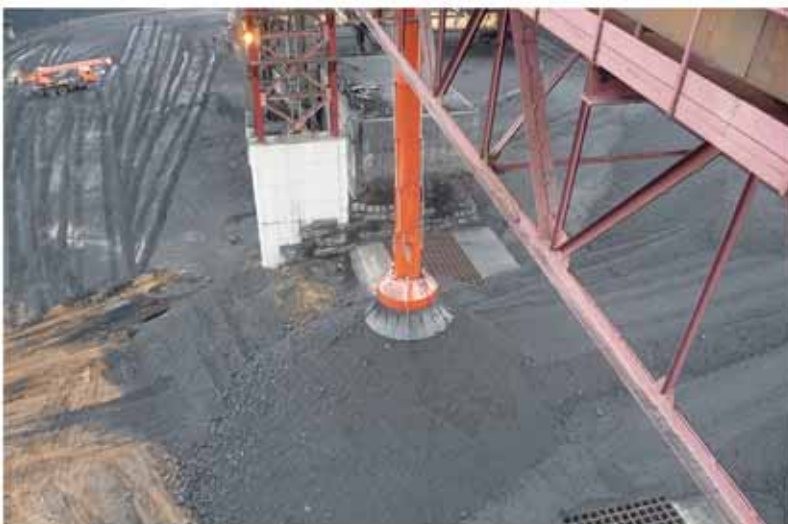
Stockpile loading spout, coal up to 450 mm, Kazakhstan
