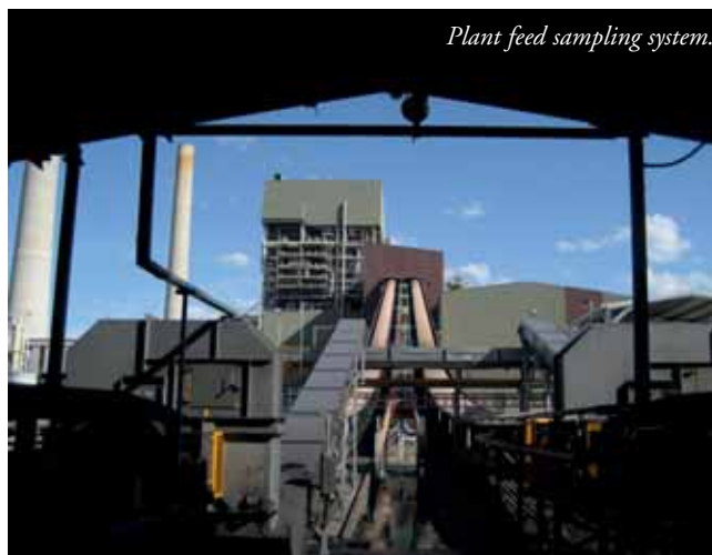
Plant feed sampling system.
