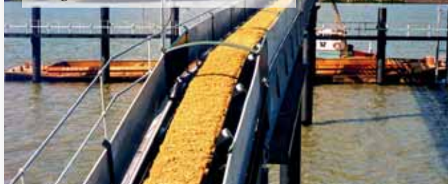
Barge loading sands and aggregates using a fixed B&W conveyor system on the River Thames, see Canary Wharf in the background under construction.
