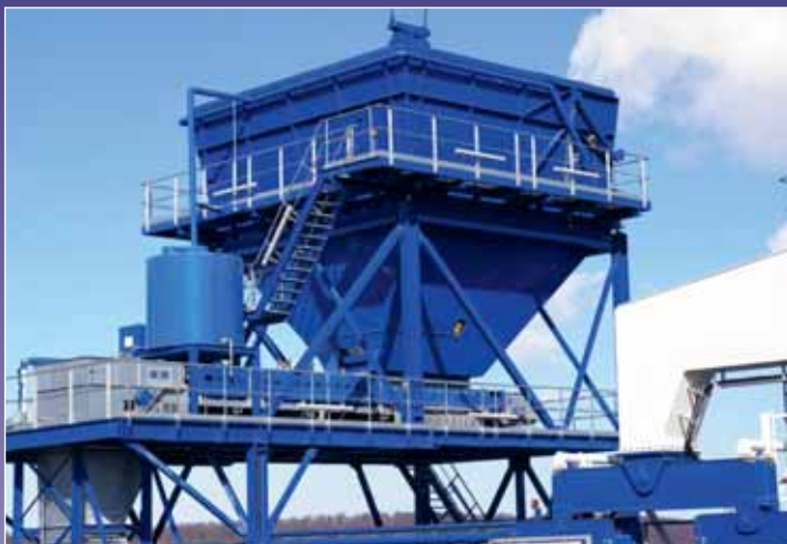
Hopper cars for ship unloading
