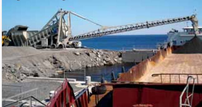
Stormajor with Samson 1600 feeder and 30m outloading boom for loading crushed stone to barges on Lake Onega in Russia.
