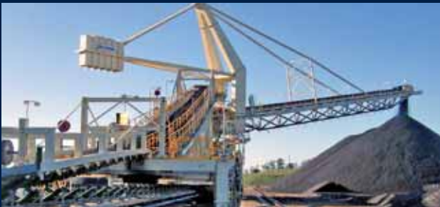
Coal Stockyard with Pylon-type Stacker
