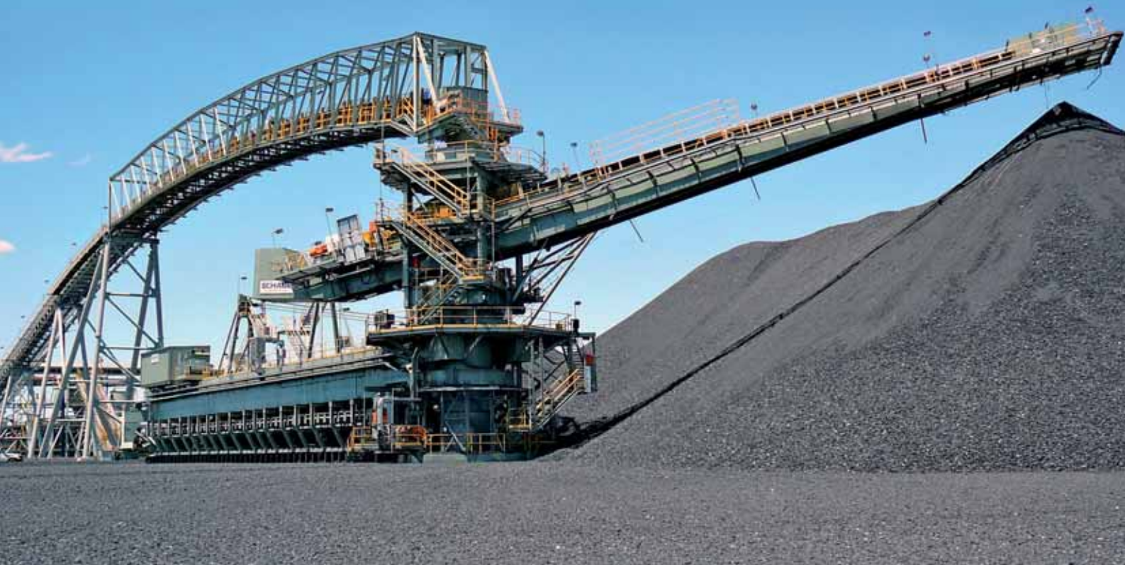
Open-air Stockyard in Coal-washing plant
