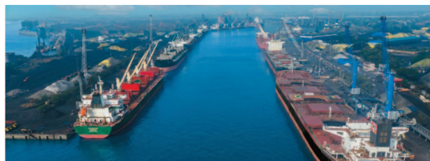
The Inner Harbour handles multiple dry cargo commodities using HMC cranes.
