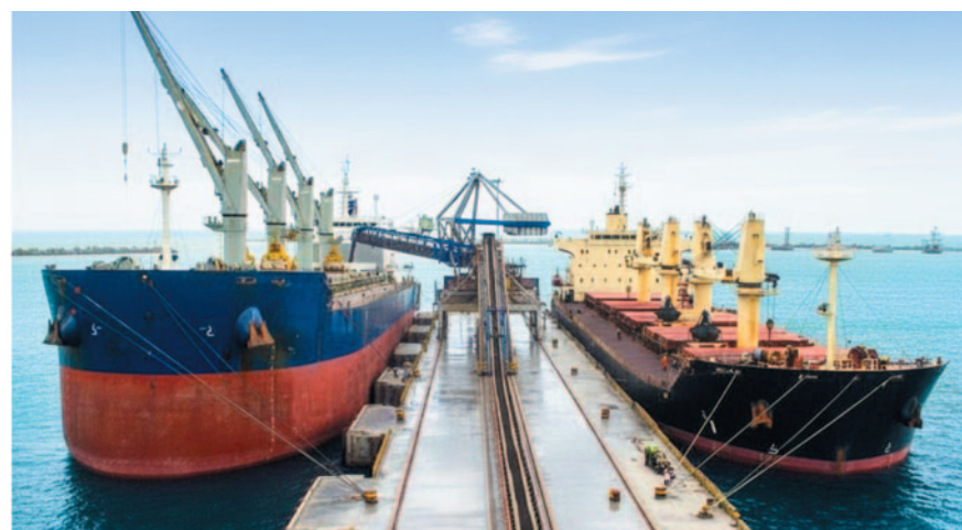
A dedicated iron ore berth is equipped with a conveyor system for efficient and continuous cargo handling.
