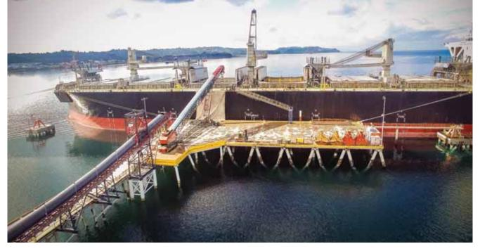
maximized along any part of the logistics chain. The investment in the TB58 Telescopic Shiploader also reduced the timeframe of the project significantly with the system fully operational in six to seven months from order.
