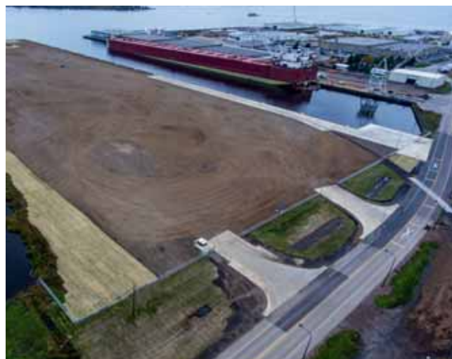
Overhead view of the newly completed 26-acre Clure Terminal Expansion, in the Port of Duluth.
