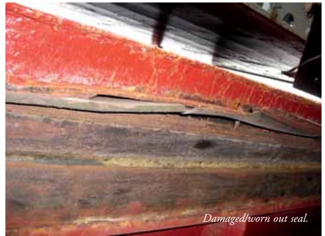
Incorrect, badly fitted repair 90°.
