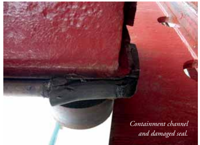
Damaged/worn out seal.
