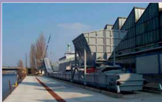
Conveying systems at the harbor
