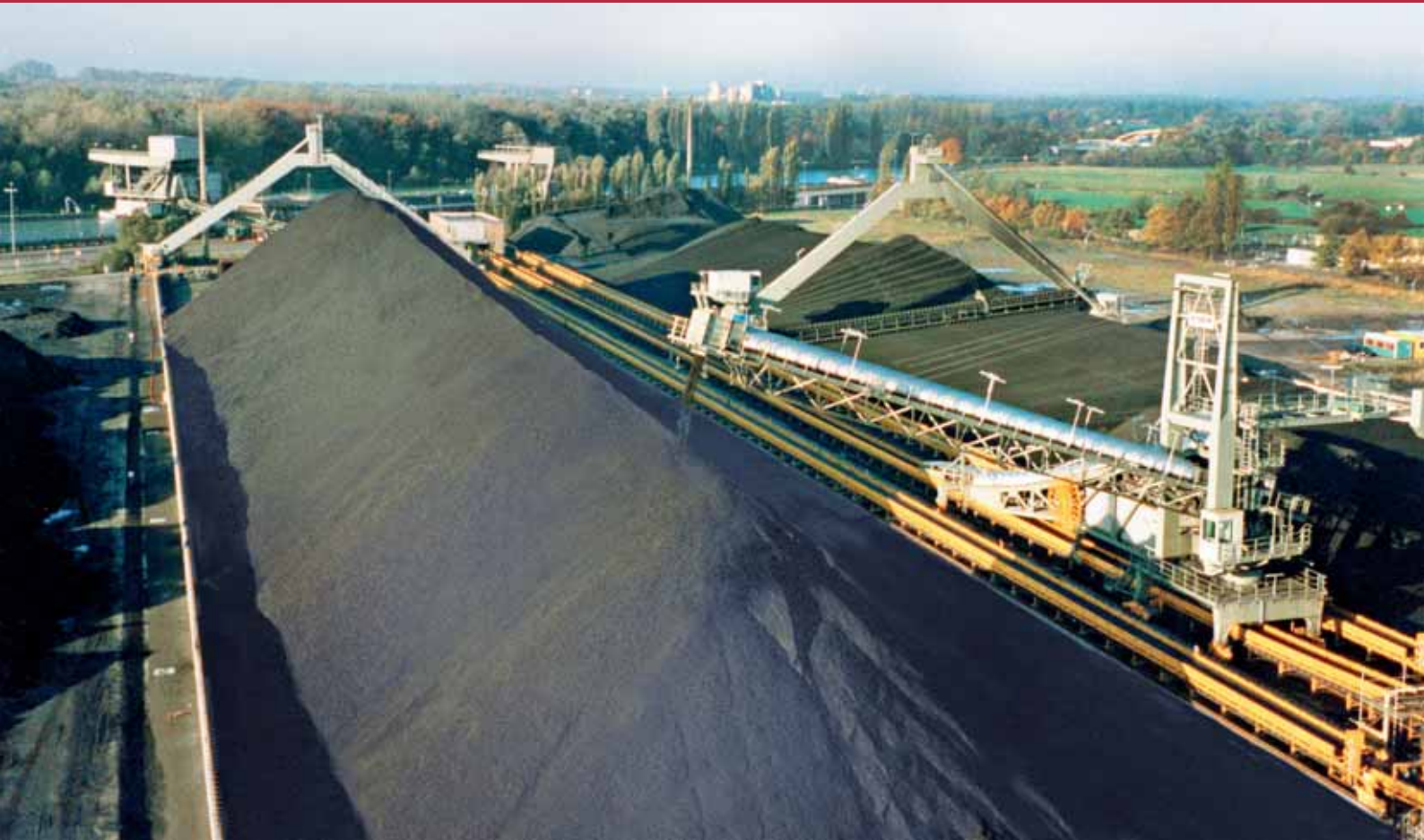
Coal Stockyard with Stacker and Portal Scraper Reclaimers
